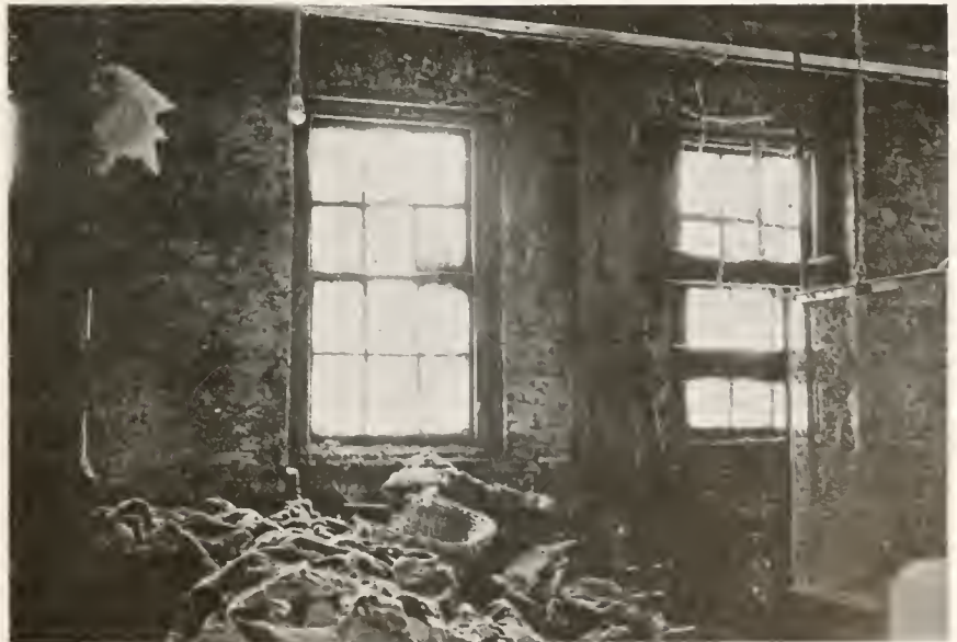
Windows of a factory found to be coated thickly with dirt and lint through which daylight was supposed to enter. After cleaning with soap and water, 29.74 per cent more light was admitted than at the time when the photograph was taken.
